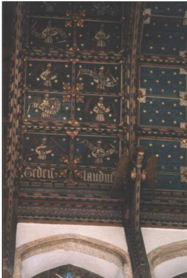
37 St. Edmund, Southwold, Suffolk. Part of the restored Roof.
