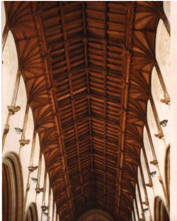
9 St. Peter Mancroft, Norwich, Norfolk. A view of the magnificent Roof showing the elaborate fan-like groining and the very long wall-posts beneath the Angels.
