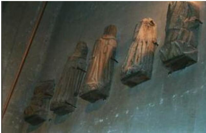
26 St. Mary, Madingley, Cambridgeshire. Damaged remnants of wooden Roof Angels.
