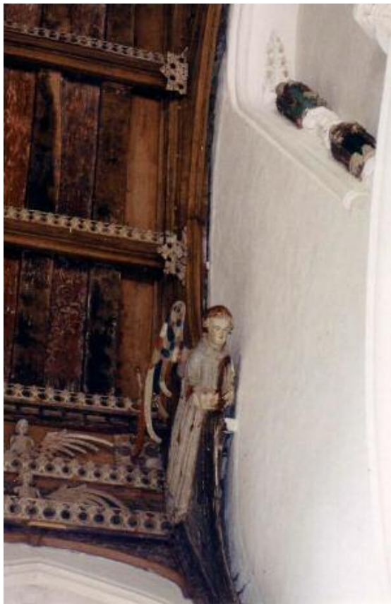
8 All Saints, Necton, Norfolk. An example of how the 15th century carpenter fitted an Angel into a tight corner by omitting to give him his second wing.
